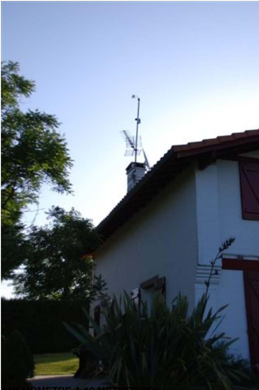
ANEMOMETRE A 10 METRES SOL
